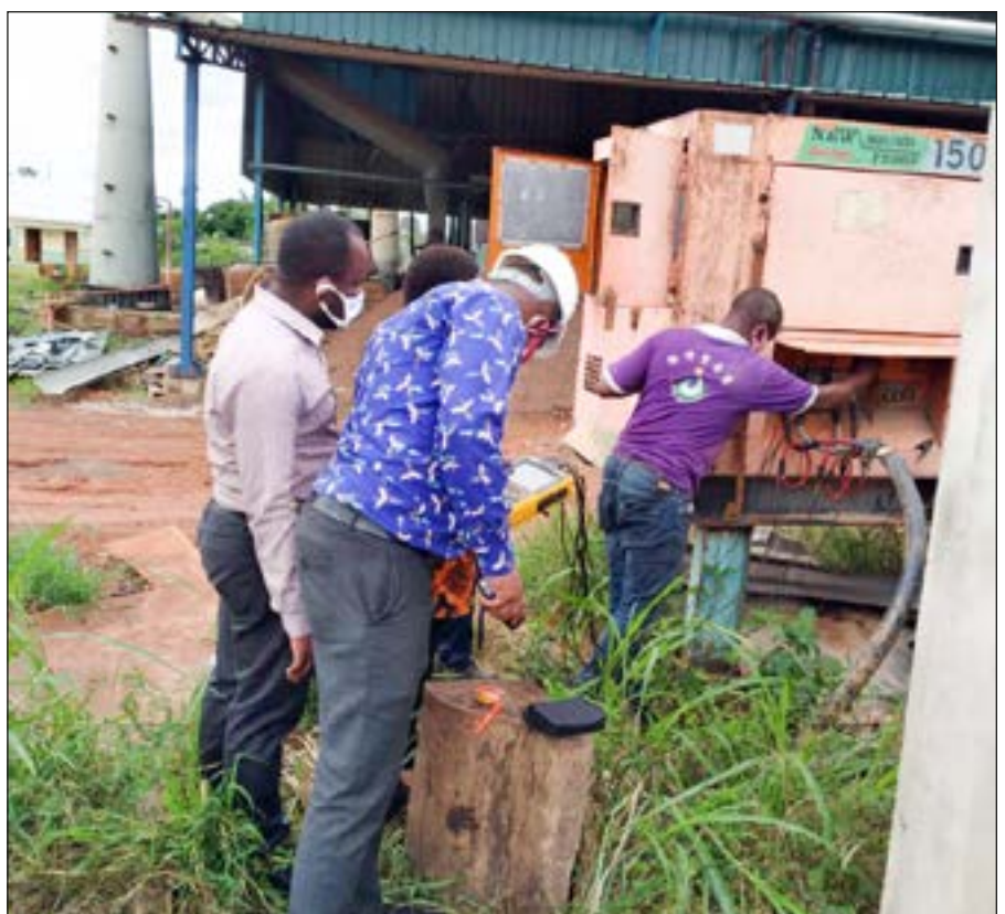
Data logging of the energy consumption of a generator plant at Vester Oil.
