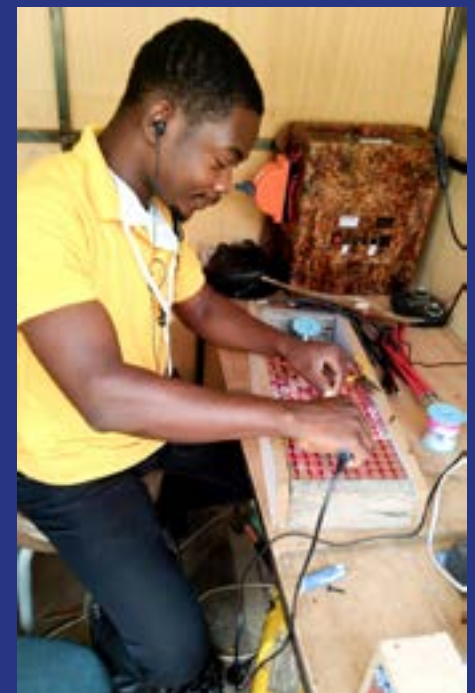
Building a 24V Lithium ion battery pack for a 5000W solar generator
