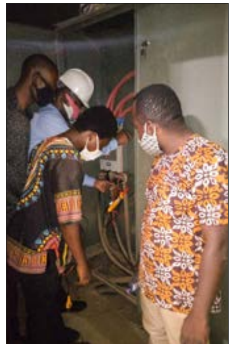
Measuring of electrical power of the systems/equipment from the main/control room
