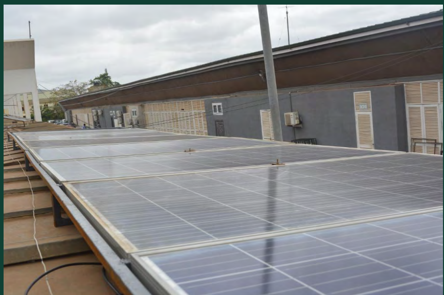
The installed solar panels
